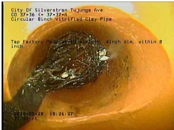
66fb8795-1478-42b5-906e-71ef41a3488f_20190528_102900_167.jpg, 00:01:09, 22.51ft Tap Factory Made at 10 o'clock, 4inch dim, within 8 inch
