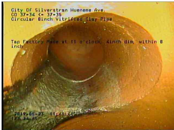
e8406855-7943-4eb3-aa26-efda9d85219e_20190523_11441_4_965.jpg, 00:12:15, 173.33ft Tap Factory Made at 11 o'clock, 4inch dim, within 8 inch
