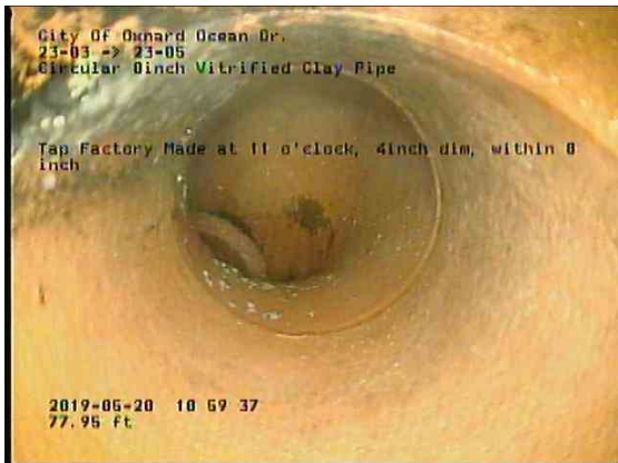
108c9e77-2afd-425b-8aa0-d59a217eebcc_20190520_110207_395.jpg, 00:05:20, 77.95ft Tap Factory Made at 11 o'clock, 4inch dim, within 8 inch
