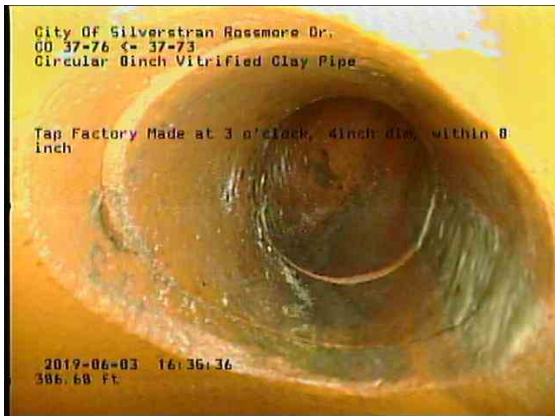
b7a76303-4fab-4f66-9d24-75a1ac8a1929_20190603_163813_754.jpg, 00:24:30, 386.68ft Tap Factory Made at 3 o'clock, 4inch dim, within 8 inch
