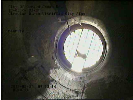
09cca0d2-3a47-41a0-8809-d4d0559fe28f_20190521_091544_486.jpg, 00:00:01, 0.00ft Manhole / 23-01
