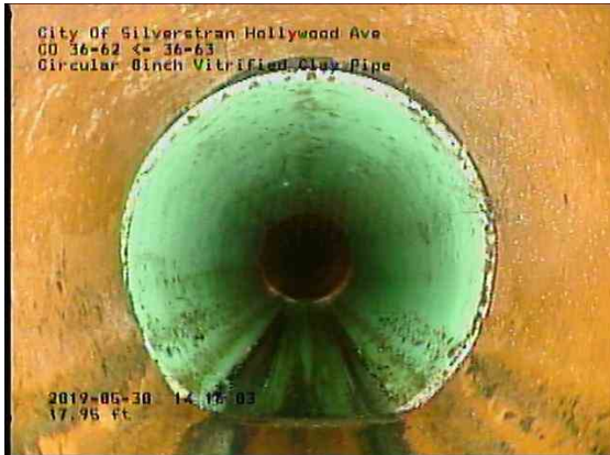
432b50fd-56a3-497e-b78c-96bd23b2d784_20190530_141839_102.jpg, 00:03:05, 18.89ft Material Change, Polyvinyl chloride / 8"
