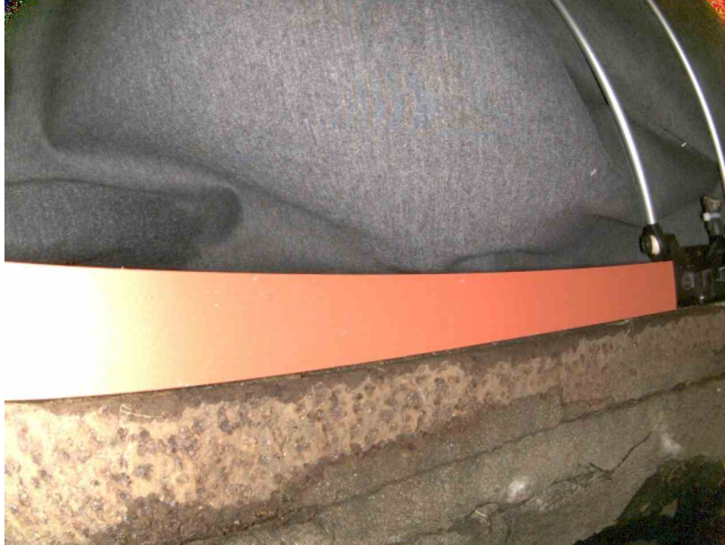
37-74-A_b7daeb13_42d1_4279_a6a1_58685002b84e_46f47148-d2d9-491e-bba8-4ebf9236c173_PL12.jpg, , -0.65 Reversal Inspection
