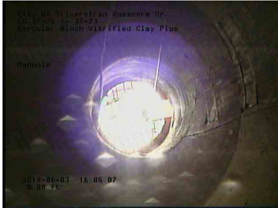
9f5ac0c5-bfdb-445a-85d8-56da139d9544_20190603_160744_204.jpg, 00:00:01, 0.00ft Manhole / 37-73
