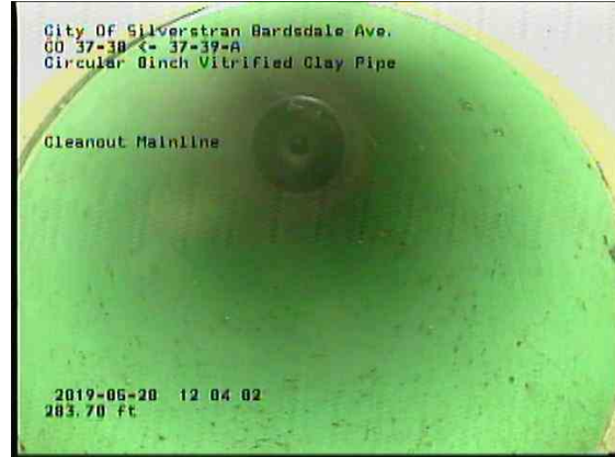
56e118c9-e897-4a89-918e-c6663c33e011_20190528_120636_057.jpg, 00:21:10, 283.70ft Cleanout Mainline / CO 37-38
