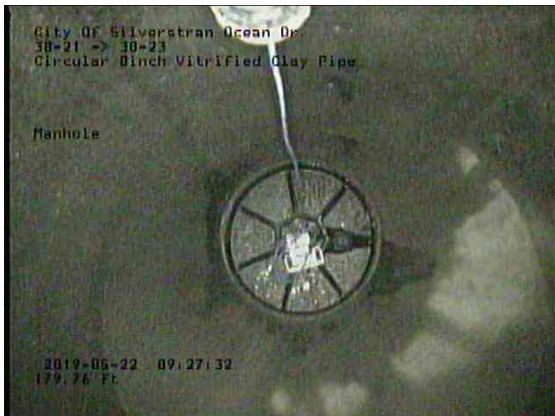
58252dd5-db5c-48a3-add8-078865523a19_20190522_093003_364.jpg, 00:11:58, 179.76ft Manhole / 38-23
