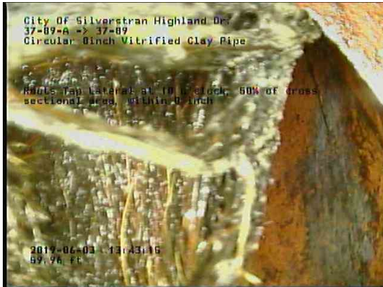
f6985a73-41b7-41fd-8bd9-a38cbefd3a78_20190603_134551_928.jpg, 00:07:58, 59.96ft Roots Tap Lateral at 10 o'clock, 50% of cross sectional area, within 8 inch
