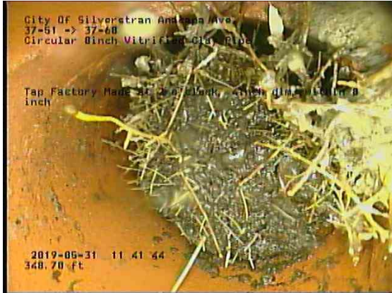
c01dee6a-7208-434c-8680-61706411ea50_20190531_114421_279.jpg, 00:21:43, 348.70ft Tap Factory Made at 2 o'clock, 4inch dim, within 8 inch
