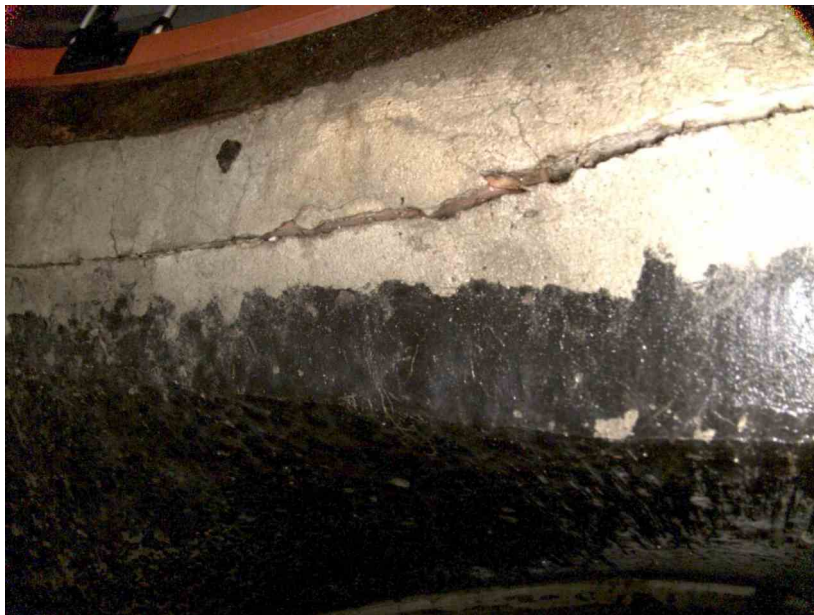
37-37-A_f72c6802_8707_4f2c_ab45_dae33749b1ef_f1bd72a2-e8fd-4bd1-b13d-6b6ee985a470_P12.jpg, , 0.31 Fracture Circumferential from 12 o'clock to 12 o'clock, within 8 inch
