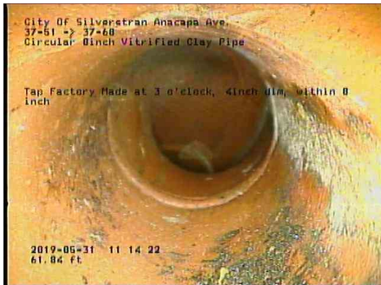
2590892c-8856-46e8-8c77-85f0256fac14_20190531_111659_497.jpg, 00:02:41, 61.83ft Tap Factory Made at 3 o'clock, 4inch dim, within 8 inch
