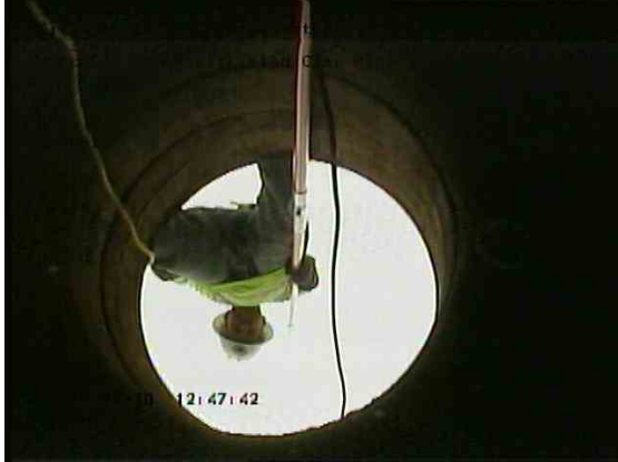
ac2367a2-1574-4609-9c6e-c54a27acdb5e_20190530_125017_336.jpg, 00:00:03, 0.00ft Manhole / 36-61
