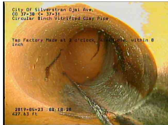
d160defc-e41b-4a27-ae26-ca5adcab7415_20190523_081301_469.jpg, 00:27:00, 427.63ft Tap Factory Made at 2 o'clock, 4inch dim, within 8 inch
