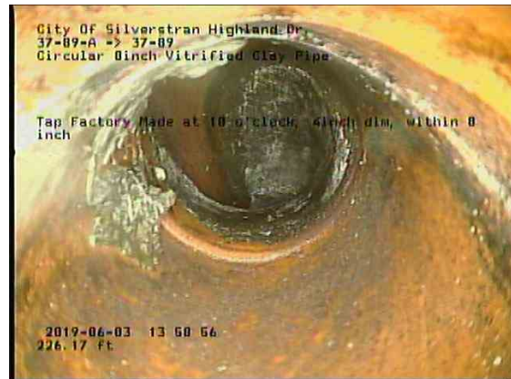
44532a31-f7ae-4aec-80c0-04df3f792ed0_20190603_140133_489.jpg, 00:21:00, 226.17ft Tap Factory Made at 10 o'clock, 4inch dim, within 8 inch
