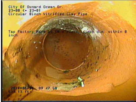
ee540337-e5d0-404c-8ac1-881e018721b3_20190521_095020_266.jpg, 00:30:18, 573.13ft Tap Factory Made at 10 o'clock, 4inch dim, within 8 inch
