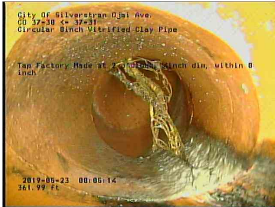
9460e475-4755-4e7d-ad16-f0a70e2f0e30_20190523_080746_617.jpg, 00:22:55, 361.99ft Tap Factory Made at 2 o'clock, 4inch dim, within 8 inch
