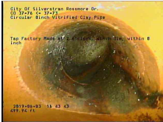
18997a62-5f79-4caa-963a-81643edfc0cb_20190603_164620_488.jpg, 00:30:54, 499.93ft Tap Factory Made at 2 o'clock, 4inch dim, within 8 inch
