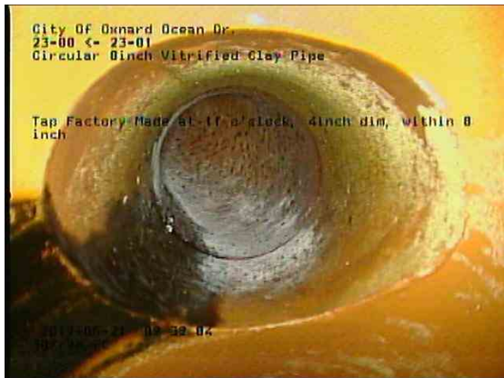
3c6a560f-d8b6-4d7a-840b-b735e9b56196_20190521_093434_276.jpg, 00:16:22, 307.94ft Tap Factory Made at 11 o'clock, 4inch dim, within 8 inch
