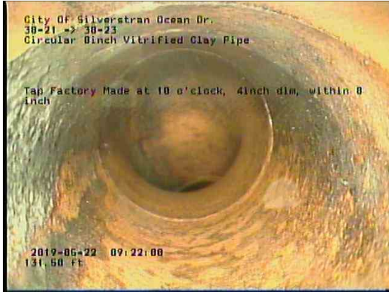
6c071ad5-744a-40a6-926b-61008a8c72a9_20190522_092431_090.jpg, 00:07:20, 131.50ft Tap Factory Made at 10 o'clock, 4inch dim, within 8 inch
