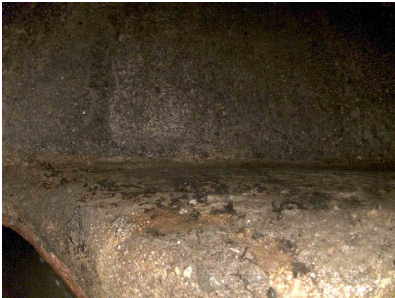
38-21_d8133f19_15ad_4f3f_8ad3_1a1fbd3e9bcc_3473cc27-aada-4e57-85ec-a1ffa681dc35_P12.jpg, , 7.04 Surface Roughness Increased at 9 o'clock, within 8 inch
