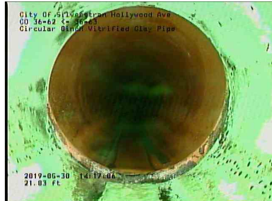
a994bc4a-7620-4bee-94f3-c3f8c21220f0_20190530_141942_075.jpg, 00:04:04, 23.33ft Material Change, Vitrified clay pipe / 8"
