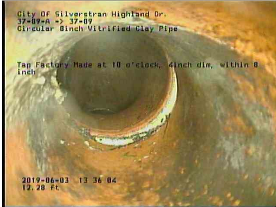
16179495-5d79-4303-bcb4-8b994807db26_20190603_133841_147.jpg, 00:03:40, 12.27ft Tap Factory Made at 10 o'clock, 4inch dim, within 8 inch
