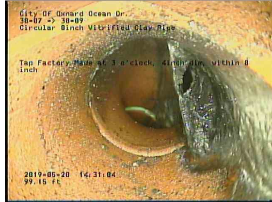
57ad780e-79de-4f49-9f73-cc6044024dd3_20190520_143334_516.jpg, 00:09:08, 99.15ft Tap Factory Made at 3 o'clock, 4inch dim, within 8 inch
