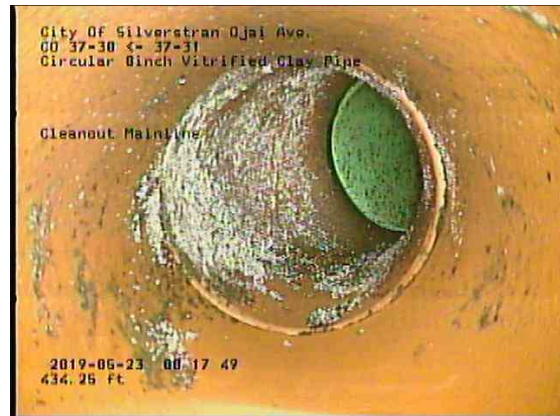
a5f464c5-e6f5-47fe-b88e-de8e7ff24372_20190523_082021_949.jpg, 00:28:17, 434.25ft Cleanout Mainline / CO 37-30
