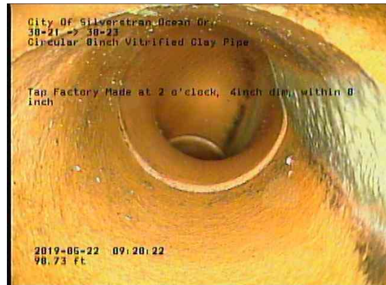
0a52ee6f-cac8-47b0-8da8-dd7701475317_20190522_092253_321.jpg, 00:05:51, 98.72ft Tap Factory Made at 2 o'clock, 4inch dim, within 8 inch
