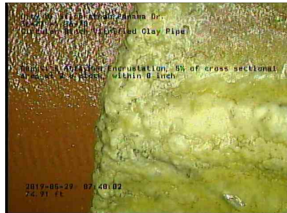
f96f1580-3a8b-4101-8529-6b99a6d25b43_20190529_074235_897.jpg, 00:04:52, 74.91ft Deposits Attached Encrustation, 5% of cross sectional area at 2 o'clock, within 8 inch
