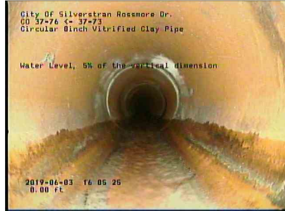
b8993029-9e58-478e-987e-a2902f9634dd_20190603_160802_931.jpg, 00:00:10, 0.00ft Water Level, 5% of the vertical dimension
