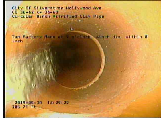
ffb0794-8991-4d2f-a3bb-3c7e26c49c29_20190530_143157_848.jpg, 00:14:37, 205.71ft Tap Factory Made at 9 o'clock, 4inch dim, within 8 inch
