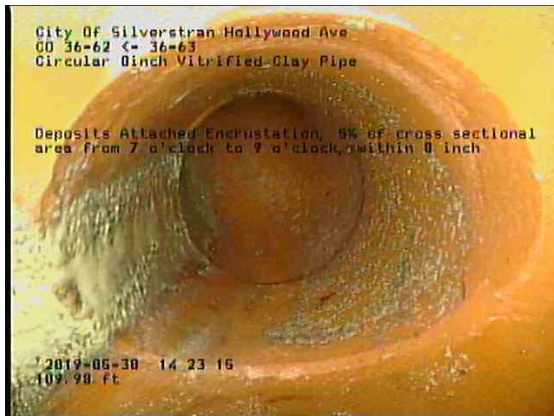
19e50abb-b200-4727-b079-6c31b828a930_20190530_142550_366.jpg, 00:09:17, 109.98ft Deposits Attached Encrustation, 5% of cross sectional area from 7 o'clock to 9 o'clock, within 8 inch / IN WYE
