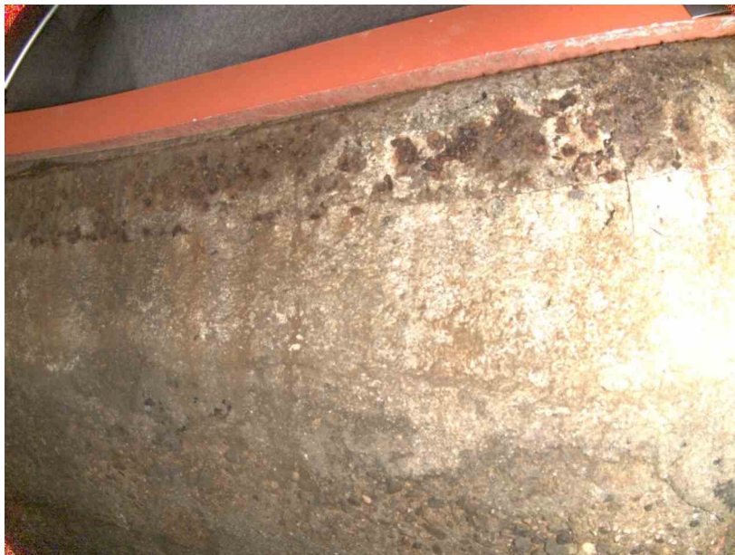
36-63_91085e16_b10b_42df_8305_4acc6363b0ef_c3bbccb1-f81e-4f4e-9064-b68c61eaf294_P12.jpg, , 0.15 Surface Roughness Increased from 12 o'clock to 12 o'clock, within 8 inch, Start
