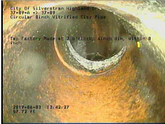
ba191ae9-f96c-454f-bc9f-53e6344cba19_20190603_134504_261.jpg, 00:07:31, 57.72ft Tap Factory Made at 2 o'clock, 4inch dim, within 8 inch
