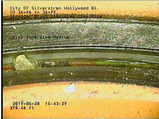
682d1afb-75bf-4c75-ab50-bdb0ab2dd5f4_20190528_154603_502.jpg, 00:15:33, 278.46ft Joint Separated Medium
