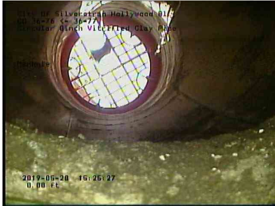
44769f0c-ed92-4ab3-9565-11518e66cfb4_20190528_152801_461.jpg, 00:00:01, 0.00ft Manhole / 36-77
