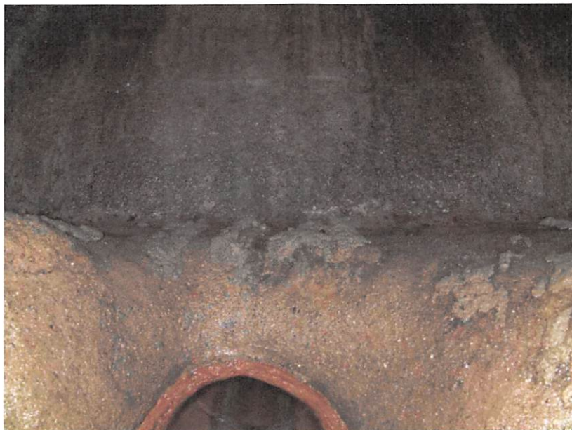
23-07_873817e9_0d4f_495f_ab7e_d928befa0923_c8057a84-4ed7-4e5c-ae3-336a8131aaed_PI2.jpg, , 7.39 Obstacles Construction Debris, 5% of cross sectional area from 11 o'clock to 3 o'clock
