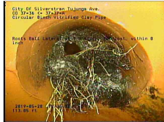
4fc087e9-805f-48db-9057-0989b8d64584_20190528_103858_389.jpg, 00:07:27, 113.05ft Roots Ball Lateral at 1 o'clock, 75% lost, within 8 inch
