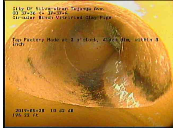
4a034020-cc42-4425-8850-ce657038de72_20190528_104513_143.jpg, 00:11:54, 196.22ft Tap Factory Made at 2 o'clock, 4inch dim, within 8 inch
