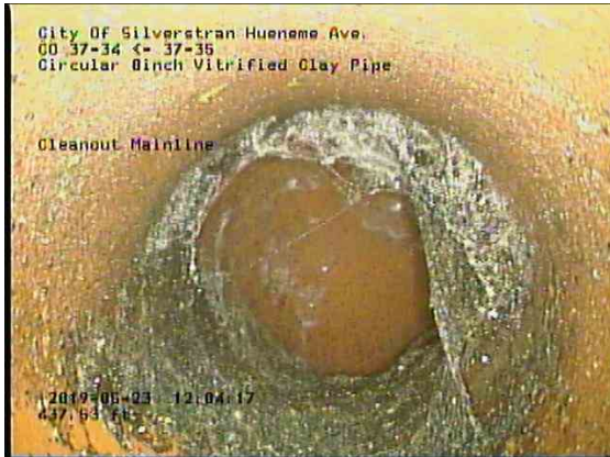
179c383c-749f-4e3d-9f00-d0941f013106_20190523_120650_460.jpg, 00:30:03, 437.53ft Cleanout Mainline / CO 37-34
