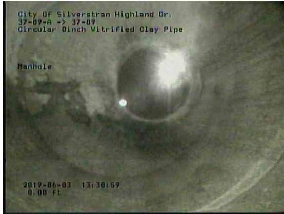
eb683f45-4487-45ec-9d1a-7fa523751da6_20190603_133336_371.jpg, 00:00:01, 0.00ft Manhole / 37-89-A
