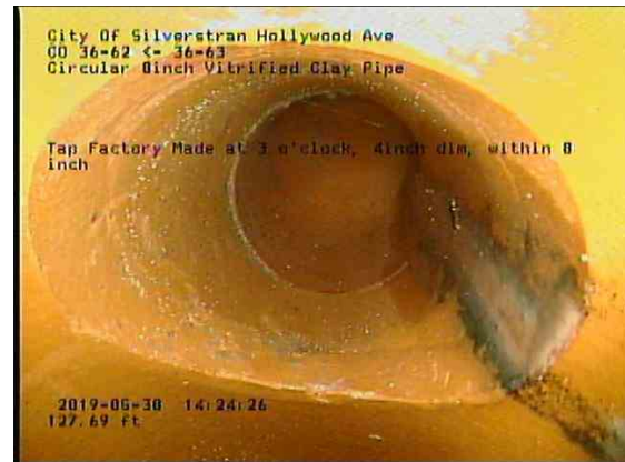
02a6d168-550f-47d4-91c3-c4b332b70f2d_20190530_142702_126.jpg, 00:10:23, 127.69ft Tap Factory Made at 3 o'clock, 4inch dim, within 8 inch
