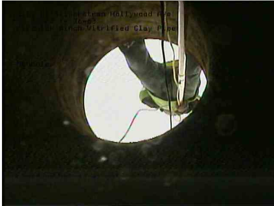
64e280de-ad57-4b70-bda5-a0b0dca5b774_20190530_140857_838.jpg, 00:00:00, 0.00ft Manhole / 36-63
