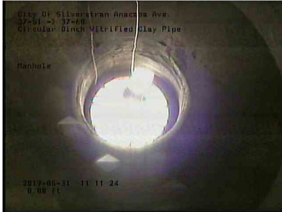
361fdffe-3bc6-4410-b54c-b61023619f64_20190531_111401_409.jpg, 00:00:01, 0.00ft Manhole / 37-51
