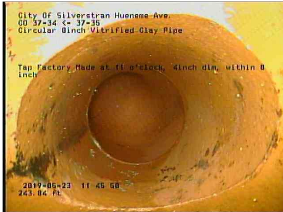
7571523a-2ee1-4807-bb71-074030b8e4c4_20190523_114823_342.jpg, 00:15:50, 243.84ft Tap Factory Made at 11 o'clock, 4inch dim, within 8 inch
