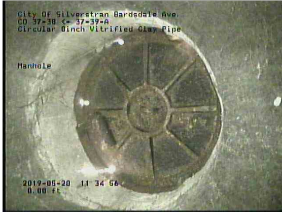
b1b9b4c0-36f7-40b9-b6ee-6683a0ce1af8_20190528_113730_446.jpg, 00:00:01, 0.00ft Manhole / 37-39-A
