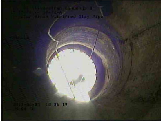
97b1fb0a-850e-4e89-a149-73ce966b87c1_20190603_102855_296.jpg, 00:00:01, 0.00ft Manhole / 37-74-A
