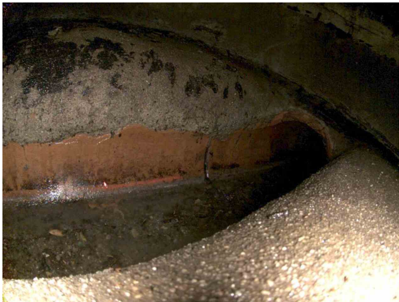
37-37-A_f72c6802_8707_4f2c_ab45_dae33749b1ef_3a91f750-6f0e-4dd4-8bfa-8dbc8c225d4f_P12.jpg, , 4.19 Surface Roughness Increased from 12 o'clock to 12 o'clock, within 8 inch
