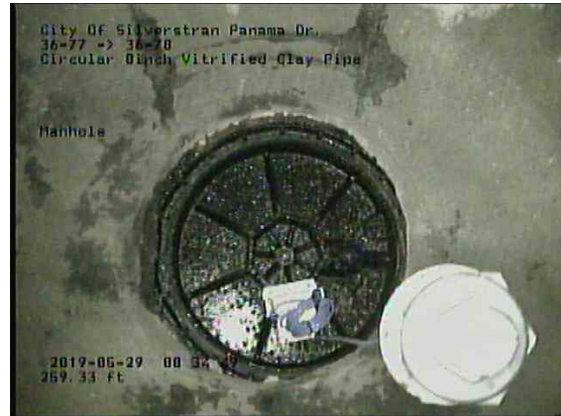
3e0b4d0f-7e60-418f-8ab6-82a98780abb1_20190529_083723_618.jpg, 00:21:25, 259.23ft Manhole / 36-78
