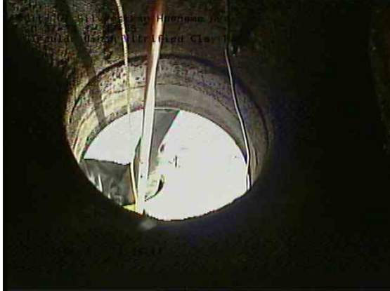
5c356c9b-47d4-4c73-a498-e345785b4da0_20190523_112644_760.jpg, 00:00:02, 0.00ft Manhole / 37-35
