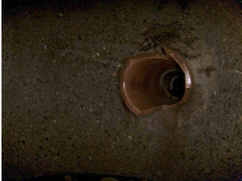
37-31_3a06f078_e941_4f01_ba58_04484b70b803_334cc57d-9868-4a8b-8237-dd6125ec6c8c_P12.jpg, , 6.14 Broken at 8 o'clock, within 8 inch
