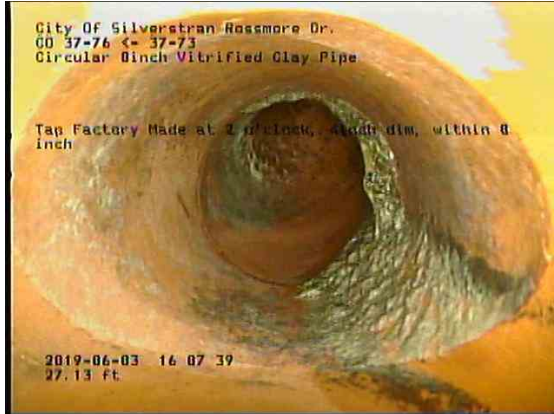
d7ee741f-2527-44a1-8e6e-b5823df3a63a_20190603_161016_254.jpg, 00:02:02, 27.13ft Tap Factory Made at 2 o'clock, 4inch dim, within 8 inch
