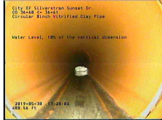
77c3219a-716f-4d37-9ef8-747b3ea9c0ad_20190530_132239_428.jpg, 00:22:51, 408.54ft Water Level, 10% of the vertical dimension
