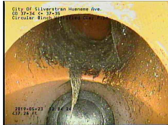
c6502d43-c4bd-4fc3-99d1-78f64c31d2fd_20190523_120657_271.jpg, 00:30:03, 437.53ft Cleanout Mainline / CO 37-34
