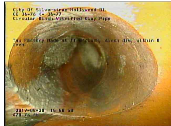
13befac9-b0a1-47d3-9231-2544b122da11_20190528_160132_363.jpg, 00:28:20, 478.74ft Tap Factory Made at 11 o'clock, 4inch dim, within 8 inch
