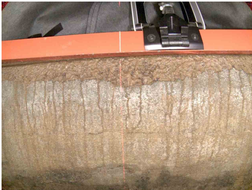
37-31_3a06f078_e941_4f01_ba58_04484b70b803_1fda0964-2329-434b-9fa4-01149b331347_P12.jpg, , 0.19 Surface Roughness Increased from 12 o'clock to 12 o'clock, within 8 inch, Start
