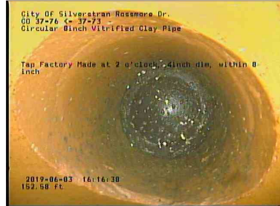
9b1fa5ce-2717-4d2b-9fd0-4c08928d8049_20190603_161915_292.jpg, 00:09:22, 152.57ft Tap Factory Made at 2 o'clock, 4inch dim, within 8 inch
