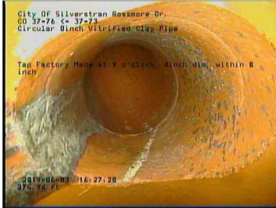
a4aa1a60-f417-4b17-88e5-2477a8ef73e8_20190603_163005_808.jpg, 00:17:37, 275.94ft Tap Factory Made at 9 o'clock, 4inch dim, within 8 inch
