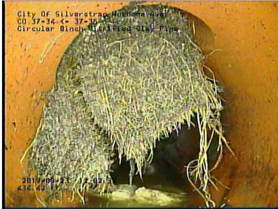
5ba93072-8966-47e2-baf5-9b7d7a0818b8_20190523_120523_5_635.jpg, 00:28:46, 434.91ft Roots Ball Lateral at 11 o'clock, 95% lost, within 8 inch
