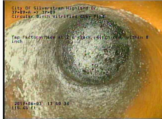
3b3ff667-4391-4bc7-bde8-f242a26f6cea_20190603_135311_586.jpg, 00:13:53, 115.45ft Tap Factory Made at 2 o'clock, 4inch dim, within 8 inch
