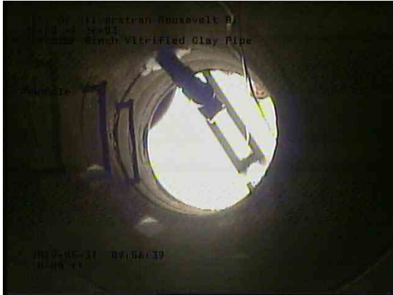
d63fcec2-bfd9-4b71-8466-26bd27e2e76d_20190531_095916_157.jpg, 00:00:00, 0.00ft Manhole / 36-82
