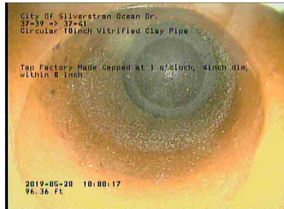
b0b65753-f8c2-4a11-810b-4ddb1f0372c_20190528_100250 _457.jpg, 00:06:48, 96.36ft Tap Factory Made Capped at 1 o'clock, 4inch dim, within 8 inch
