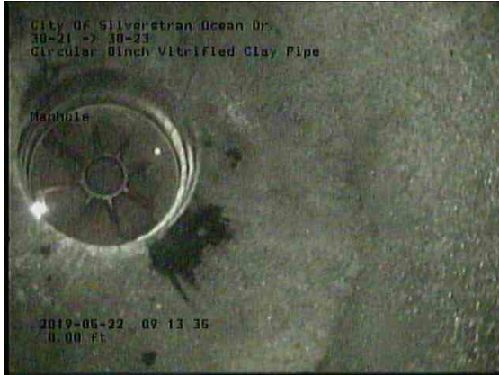
79228577-f8b4-4968-81d1-13dd78ca4f5d_20190522_091606_444.jpg, 00:00:03, 0.00ft Manhole / 38-21
