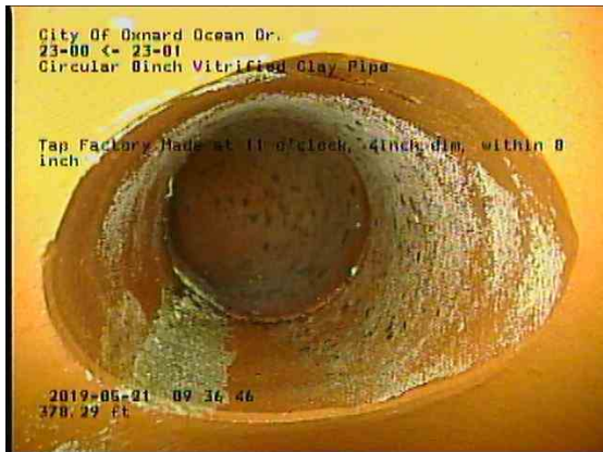
27dca17a-b142-4ee4-a522-cda820e102e0_20190521_093915_962.jpg, 00:20:28, 378.29ft Tap Factory Made at 11 o'clock, 4inch dim, within 8 inch
