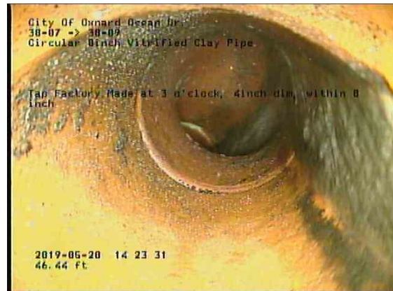
c77ec91d-1de4-43ef-8a3a-fef08d21938e_20190520_142601_386.jpg, 00:04:17, 46.44ft Tap Factory Made at 3 o'clock, 4inch dim, within 8 inch
