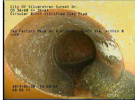
cca830bf-5c03-4015-b2e6-b78b8586f403_20190530_130130_011.jpg, 00:05:32, 68.85ft Tap Factory Made at 2 o'clock, 4inch dim, within 8 inch
