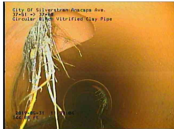
68e3838c-b496-4fec-b6a1-7136f665705c_20190531_114140_110.jpg, 00:20:41, 346.00ft Roots Medium Lateral at 11 o'clock, 45% lost
