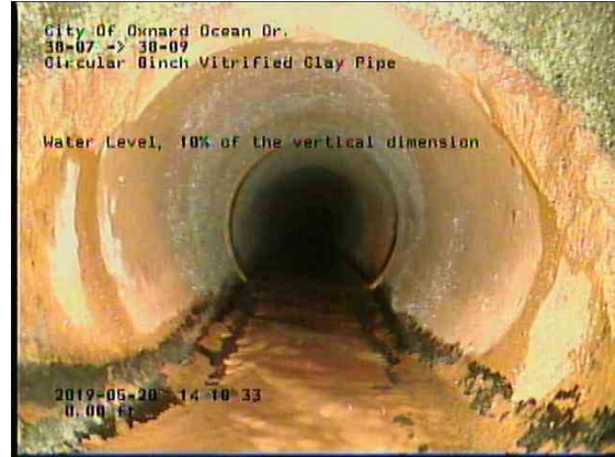
63071976-97b0-4a3a-8a6a-2794165f44ad_20190520_142110_3_512.jpg, 00:00:10, 0.00ft Water Level, 10% of the vertical dimension
