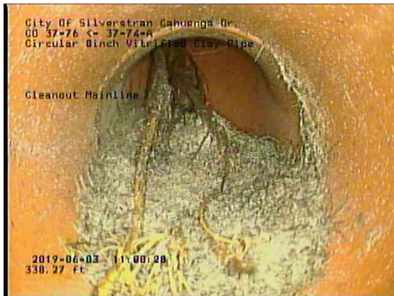
e053d589-aa6e-4a65-b538-23ca1252f971_20190603_110304_401.jpg, 00:23:08, 338.27ft Cleanout Mainline / CO 37-76
