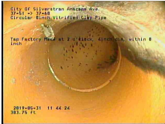
9690bd7d-358e-4d52-8c2c-168410059ebc_20190531_114701_010.jpg, 00:23:53, 383.75ft Tap Factory Made at 2 o'clock, 4inch dim, within 8 inch
