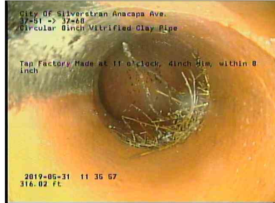
93b2db1f-00a0-49d8-870b-6cc61bf12bf2_20190531_113833_606.jpg, 00:18:47, 316.02ft Tap Factory Made at 11 o'clock, 4inch dim, within 8 inch
