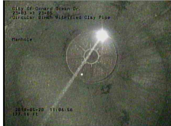
b175dbbf-c158-4ebe-aaf6-bd43f2032594_20190520_110926_087.jpg, 00:11:41, 177.16ft Manhole / 23-05
