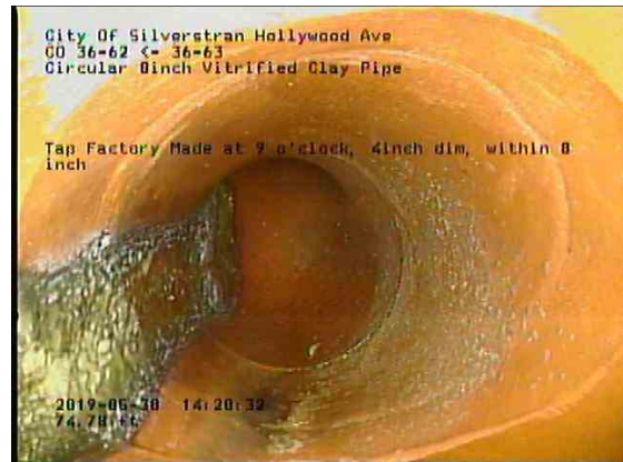
cc98de8e-d84c-4018-b2e1-8fa95cc768f5_20190530_142307_305.jpg, 00:07:11, 74.78ft Tap Factory Made at 9 o'clock, 4inch dim, within 8 inch
