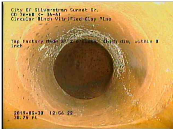
608a5b8a-ae07-43d8-82a4-b4dd4863963e_20190530_125858_024.jpg, 00:03:30, 38.75ft Tap Factory Made at 2 o'clock, 4inch dim, within 8 inch
