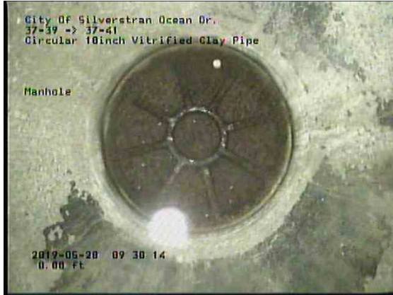
897d14b4-dd8d-44f9-a575-712ac9c12477_20190528_094047_582.jpg, 00:00:01, 0.00ft Manhole / 37-39
