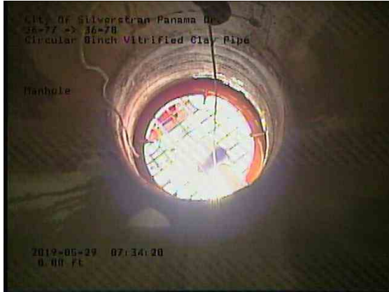
319936ff-3168-4ee2-94d6-238c697c1a84_20190529_073654_453.jpg, 00:00:00, 0.00ft Manhole / 36-77
