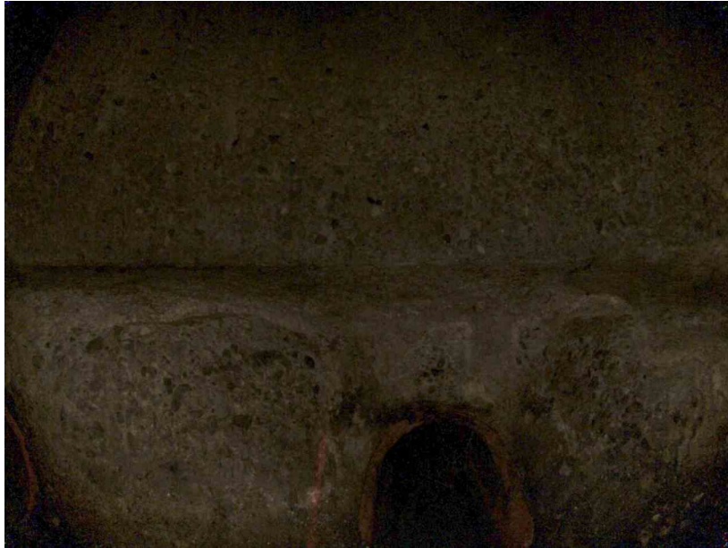
23-03_caf8412c_d397_4fc6_88c9_a9658e397a0b_6e0396ac-f9fa-4104-9d2d-3f46652794dd_P12.jpg, , 6.75 Surface Aggregate Visible, from 07 to -01 o'clock, within 8 inch
