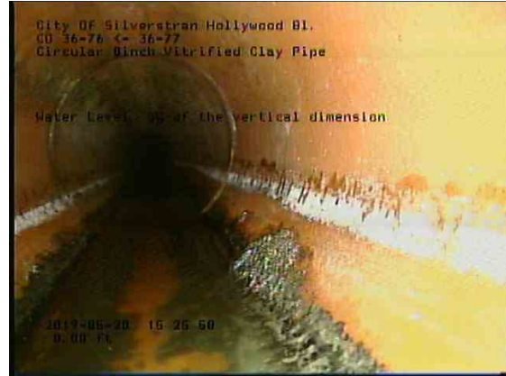
7e3d7280-e8e0-429c-b15d-552f88a09e9c_20190528_152824_776.jpg, 00:00:16, 0.00ft Water Level, 5% of the vertical dimension
