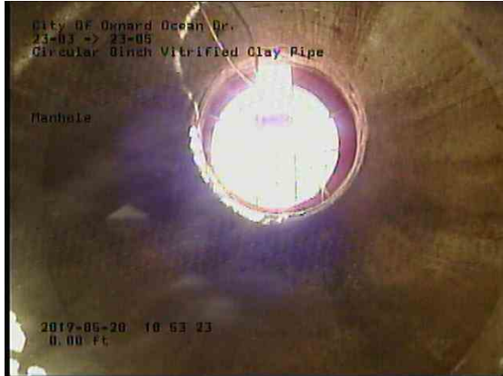
bd29e82a-fd79-48ab-b537-993bf6e9d478_20190520_105552_672.jpg, 00:00:01, 0.00ft Manhole / 23-03
