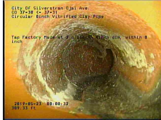
7ba14894-fed3-43ac-b0b1-0c6ee8bbbb7c_20190523_080304_590.jpg, 00:19:12, 309.33ft Tap Factory Made at 2 o'clock, 4inch dim, within 8 inch
