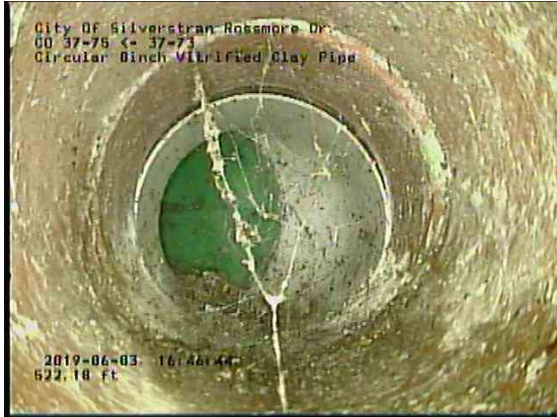
8087cb28-8337-4831-8af3-b49e2e288916_20190603_164921_847.jpg, 00:32:43, 522.18ft Cleanout Mainline / CO 37-75
