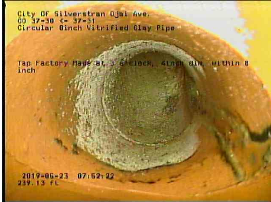
92fb7d03-03bd-4922-978f-05b955276836_20190523_075454_741.jpg, 00:14:12, 239.13ft Tap Factory Made at 3 o'clock, 4inch dim, within 8 inch
