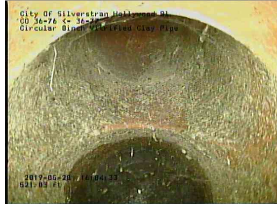
0dd623af-c7e7-4d8f-9e6f-198fb7e8fcad_20190528_160707_458.jpg, 00:31:41, 521.27ft Cleanout Mainline / CO 36-76
