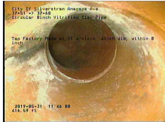
add5b87d-43cb-4576-84c7-78eb8cce85de_20190531_114837_535.jpg, 00:25:23, 416.59ft Tap Factory Made at 11 o'clock, 4inch dim, within 8 inch
