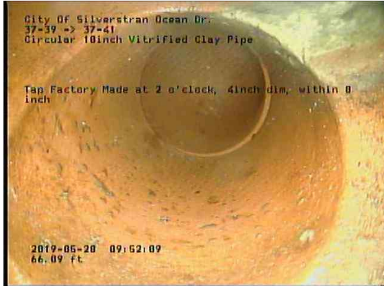
e363a8fb-1508-429d-9370-07233e3a1b85_20190528_09544 2_749.jpg, 00:05:14, 66.09ft Tap Factory Made at 2 o'clock, 4inch dim, within 8 inch
