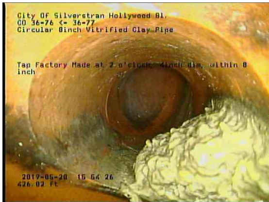
a7c3c2fb-e00d-4219-a847-f17be3de891f_20190528_155701_020.jpg, 00:25:02, 426.02ft Tap Factory Made at 2 o'clock, 4inch dim, within 8 inch
