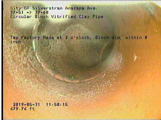
314ca382-5f43-48f3-b57f-1c2692ed61ce_20190531_115252_668.jpg, 00:28:37, 479.63ft Tap Factory Made at 2 o'clock, 8inch dim, within 8 inch
