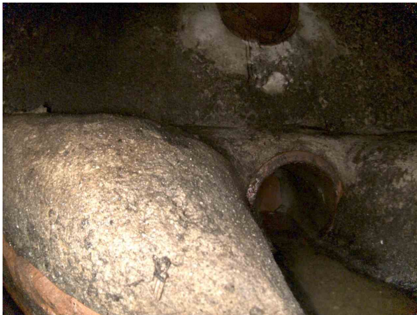
36-61_cd22f785_8cc2_4e9f_ab8d_76fe60c0a5c6_f975e6f6-4e51-4e4c-85ba-067451ce1c57_P12.jpg, , 6.57 Surface Roughness Increased from 12 o'clock to 12 o'clock, within 8 inch, Finish
