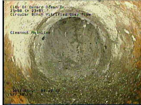
17c3c5be-0d45-4d38-b486-097a7ec0c484_20190521_095117_149.jpg, 00:30:58, 577.68ft Cleanout Mainline / CO 8"
