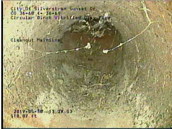
f689bf3c-7808-423e-aa57-2ddca0096b46_20190530_133228_231.jpg, 00:29:57, 518.07ft Cleanout Mainline / CO 36-60
