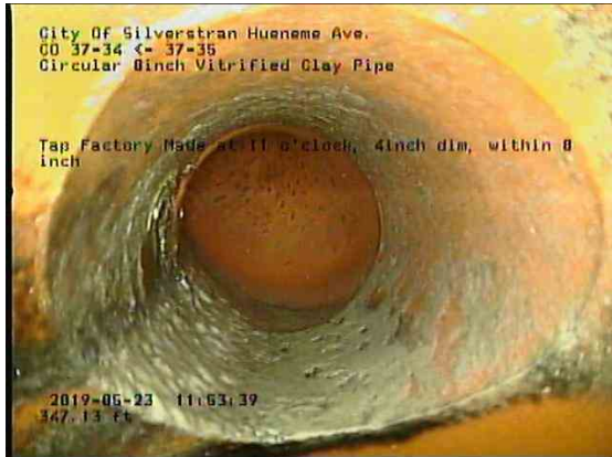
edd47f34-6887-49b1-8ece-c525b15464cb_20190523_115612_059.jpg, 00:21:44, 347.13ft Tap Factory Made at 11 o'clock, 4inch dim, within 8 inch
