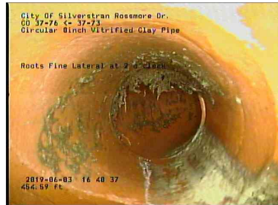
c412fb7a-02bc-4c85-b192-9c22b41fb58e_20190603_164314_588.jpg, 00:28:27, 454.59ft Roots Fine Lateral at 2 o'clock
