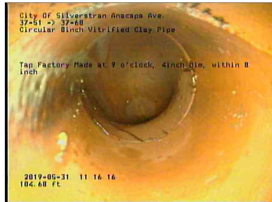
5b5602b9-a745-4152-b46e-18344f101362_20190531_111853_466.jpg, 00:04:29, 104.68ft Tap Factory Made at 9 o'clock, 4inch dim, within 8 inch
