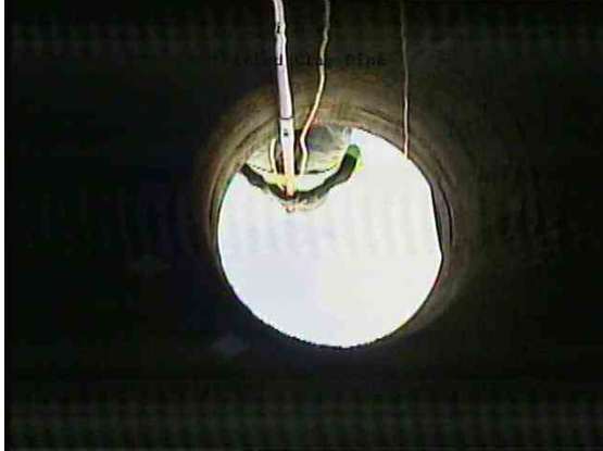
b683247e-4f74-46ca-aac8-afcf11130179_20190523_072412_414.jpg, 00:00:01, 0.00ft Manhole / 37-31
