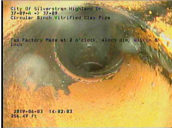
11865b35-195b-4b69-b9bf-9ba092ea9eb4_20190603_140440_127.jpg, 00:23:20, 256.49ft Tap Factory Made at 2 o'clock, 4inch dim, within 8 inch
