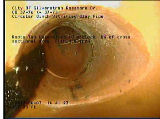
a827ff68-0464-49df-b5ad-0c2ef7003cc0_20190603_164400_767.jpg, 00:28:52, 457.23ft Roots Tap Lateral at 10 o'clock, 5% of cross sectional area, within 8 inch
