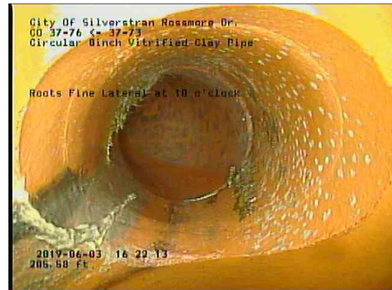
69f70465-a8ea-465d-8c1f-9d0bea1e34c9_20190603_162450_262.jpg, 00:13:25, 205.58ft Roots Fine Lateral at 10 o'clock
