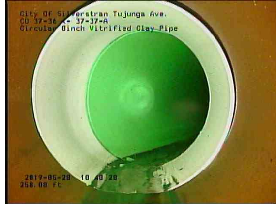
8f57d2ac-fd55-4ccb-b94a-9f62597bfbb3_20190528_105101_705.jpg, 00:15:53, 258.65ft Material Change, Polyvinyl chloride / 8"
