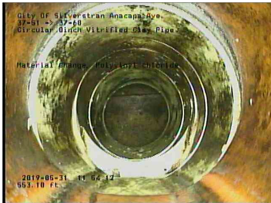
d272b511-7f50-417a-8d1b-1b3ea1bf7a0d_20190531_115649_715.jpg, 00:32:47, 554.02ft Material Change, Polyvinyl chloride / 8"
