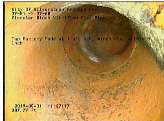
387cbcae-f37e-4eac-8d32-d4b4d9aa829d_20190531_112954_767.jpg, 00:12:08, 207.77ft Tap Factory Made at 1 o'clock, 4inch dim, within 8 inch
