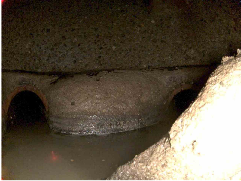
37-31_3a06f078_e941_4f01_ba58_04484b70b803_5df3d54f-4224-42d2-af69-956cb8b554bf_P12.jpg, , 8.18 Surface Roughness Increased from 12 o'clock to 12 o'clock, within 8 inch, Finish
