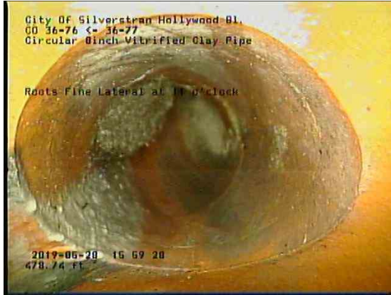
6786af43-bce4-412f-a4cd-55417416a8a7_20190528_160203_025.jpg, 00:28:23, 478.74ft Roots Fine Lateral at 11 o'clock
