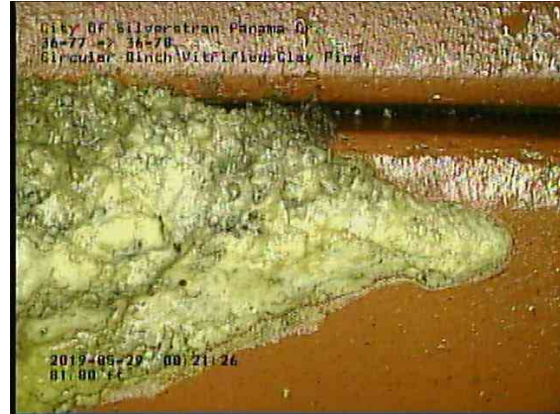
55ca7758-bb11-4754-8199-1bfd5d77443b_20190529_082400_682.jpg, 00:09:22, 81.80ft Deposits Attached Encrustation, 5% of cross sectional area from 7 o'clock to 10 o'clock, within 8 inch
