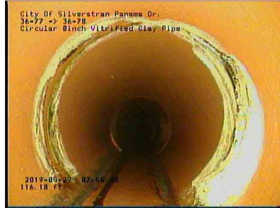
270999aa-7fa8-452d-a0dc-ac5f1411e198_20190529_075814_273.jpg, 00:13:44, 117.39ft Deposits Attached Encrustation, 5% of cross sectional area from 8 o'clock to 4 o'clock, within 8 inch
