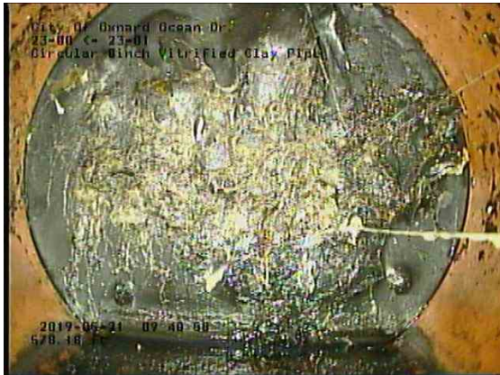
760c0f61-6c36-47fa-ba4d-1e2d8f7532b9_20190521_095128_698.jpg, 00:30:58, 577.68ft Cleanout Mainline / CO 8"
