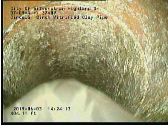
896d838c-f4f8-4abe-843e-670fcf431432_20190603_142649_878.jpg, 00:36:47, 404.11ft Tee Connection at 6 o'clock, 8"inch vertical, 8"inch horizontal / DROP
