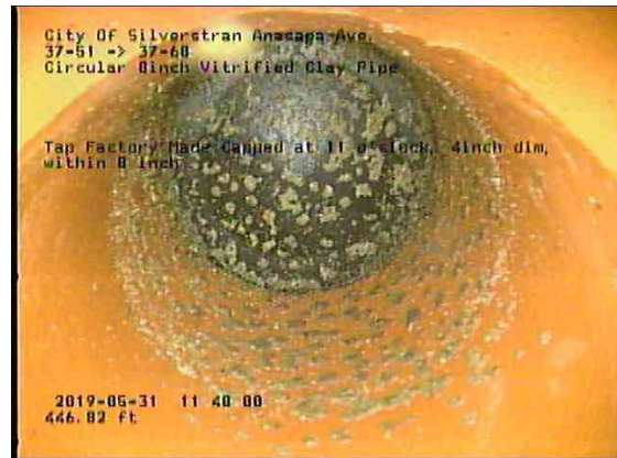
21ccb82c-7e48-4219-bcc9-5561d53def3d_20190531_115037_122.jpg, 00:27:05, 446.82ft Tap Factory Made Capped at 11 o'clock, 4inch dim, within 8 inch
