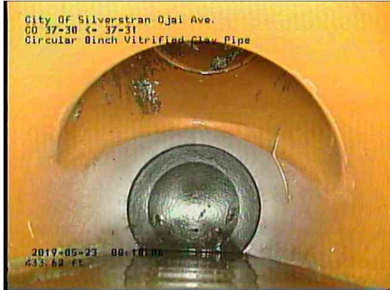
7aad6f1d-95e7-4ec0-a1a8-414c14f8c020_20190523_082038_809.jpg, 00:28:17, 434.25ft Cleanout Mainline / CO 37-30
