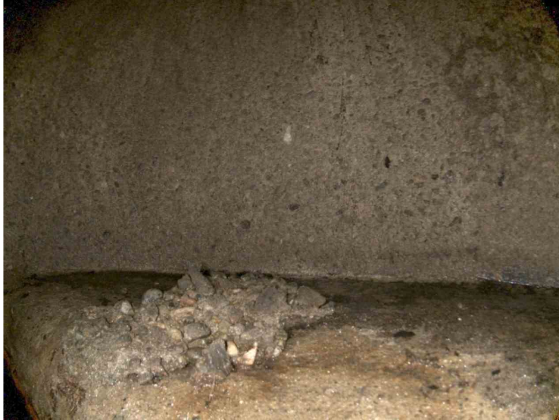
37-89-A_b79949af_46fc_4028_94b0_26ae49ec5641_ecc5a2b4-0e5d-4a59-bd74-3ad261f44915_P12.jpg, , 9.65 Deposits Settled Compacted, 5% of cross sectional area at 1 o'clock, within 8 inch
