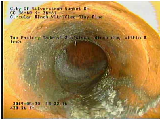
697172dd-3538-448d-a8f7-a92a844c28ff_20190530_132425_014.jpg, 00:24:23, 438.26ft Tap Factory Made at 2 o'clock, 4inch dim, within 8 inch
