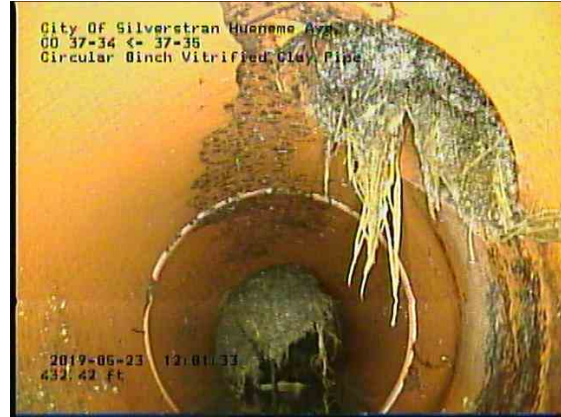
9337195d-4944-4e3e-a0c4-26838f119cc5_20190523_120406_237.jpg, 00:27:58, 432.71ft Roots Ball Lateral from 1 o'clock to 2 o'clock, 90% lost, within 8 inch
