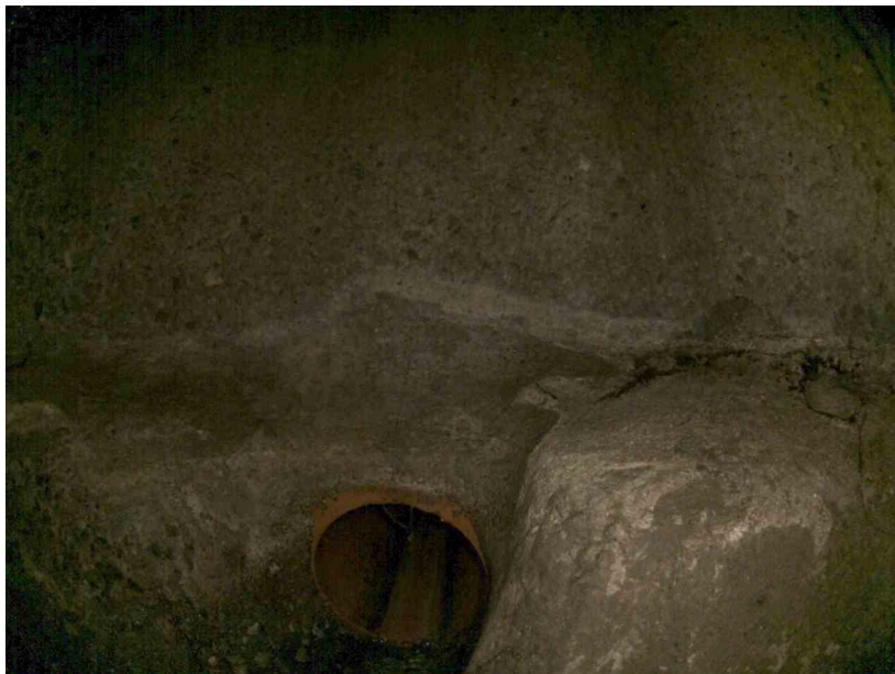
23-03_caf8412c_d397_4fc6_88c9_a9658e397a0b_9db6ab04-c3ca-44fc-92b4-d1dbc7caf386_P12.jpg, , 6.20 Surface Roughness Increased, from 10 to -01 o'clock, within 8 inch, F01
