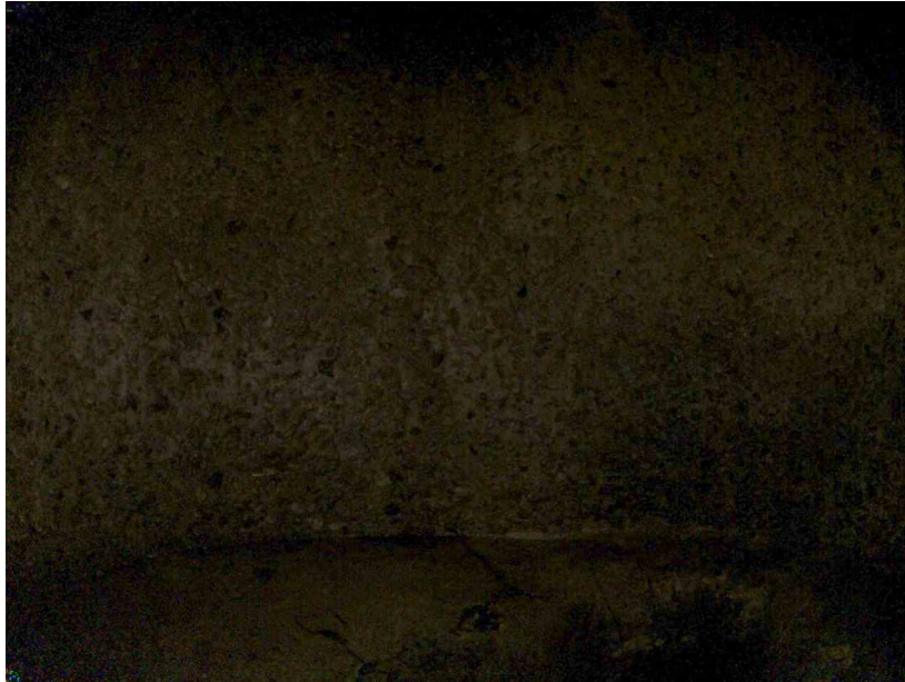
23-05_07f89197_7dd0_4207_a0d5_4ab641627b63_a570f22f-c49a-46ac-ab6d-dea4decc156f_P12.jpg, , 5.88 Surface Aggregate Visible from 3 o'clock to 6 o'clock, within 8 inch
