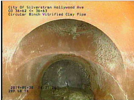
7b6a12f0-1c62-44f8-8f06-2aa9fbd34e26_20190530_143401_430.jpg, 00:15:27, 210.59ft Cleanout Mainline / CO 36-62
