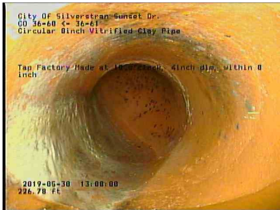
dff59292-d493-496e-aa78-4e3a117aef4d_20190530_131035_593.jpg, 00:13:00, 226.78ft Tap Factory Made at 10 o'clock, 4inch dim, within 8 inch
