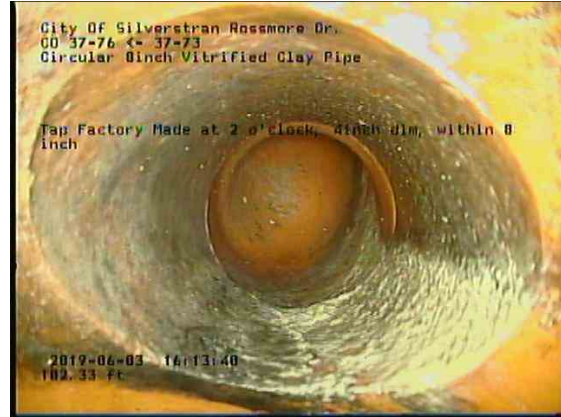
bdf539d2-c24b-4abc-abc6-66844ede13c5_20190603_161617_142.jpg, 00:06:52, 102.33ft Tap Factory Made at 2 o'clock, 4inch dim, within 8 inch
