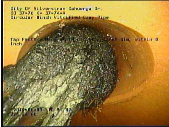
9bcdd12f-cf9b-457a-8f16-5183a2424d03_20190603_105345_308.jpg, 00:17:48, 276.24ft Tap Factory Made at 10 o'clock, 4inch dim, within 8 inch
