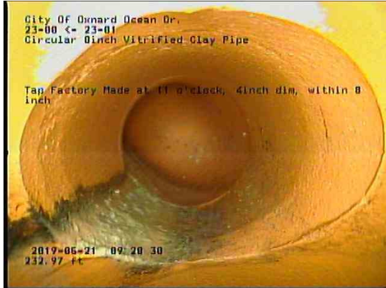
e791b170-c8d1-46fa-b199-d18a7556fdc0_20190521_093100_846.jpg, 00:13:06, 232.97ft Tap Factory Made at 11 o'clock, 4inch dim, within 8 inch
