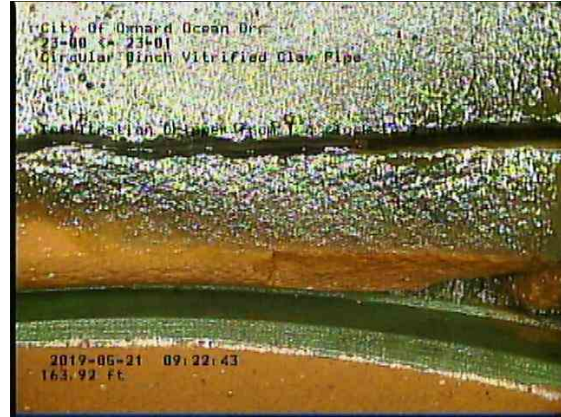
959fd213-f6cf-4cdb-a641-d7b32facfca_20190521_092513_286.jpg, 00:08:13, 163.92ft Infiltration Dripper from 1 o'clock to 2 o'clock
