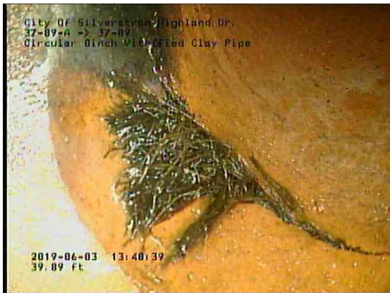
b9d023d2-ed2e-4098-8b53-f45bd66af059_20190603_134316_211.jpg, 00:05:57, 39.85ft Roots Fine Lateral at 10 o'clock
