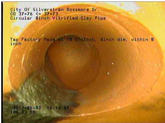
9ca10b98-cd41-4ef9-a4d2-854d5cc6ec9c_20190603_161645_045.jpg, 00:07:12, 104.82ft Tap Factory Made at 10 o'clock, 4inch dim, within 8 inch
