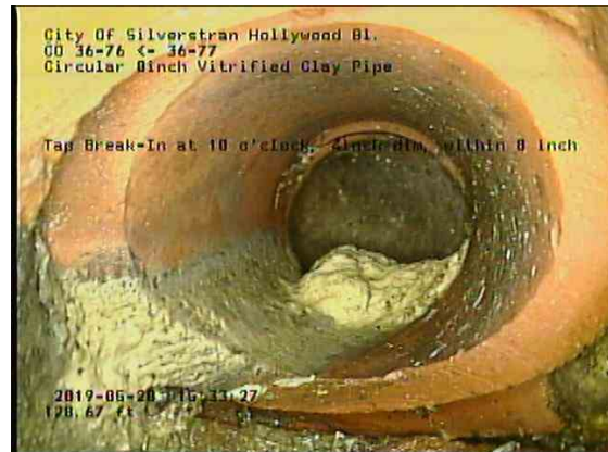
ff2d22fc-bded-4ae6-8ace-156620135091_20190528_153601_986.jpg, 00:07:03, 128.67ft Tap Break-In at 10 o'clock, 4inch dim, within 8 inch
